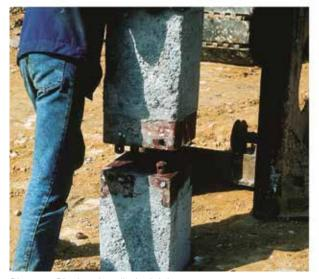
Phase 1: Placing the pile for joining
