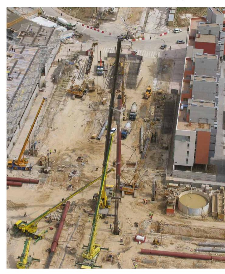
More than 500.000 m2 of diaphragm wall carried out by using Trench Cutter technique
